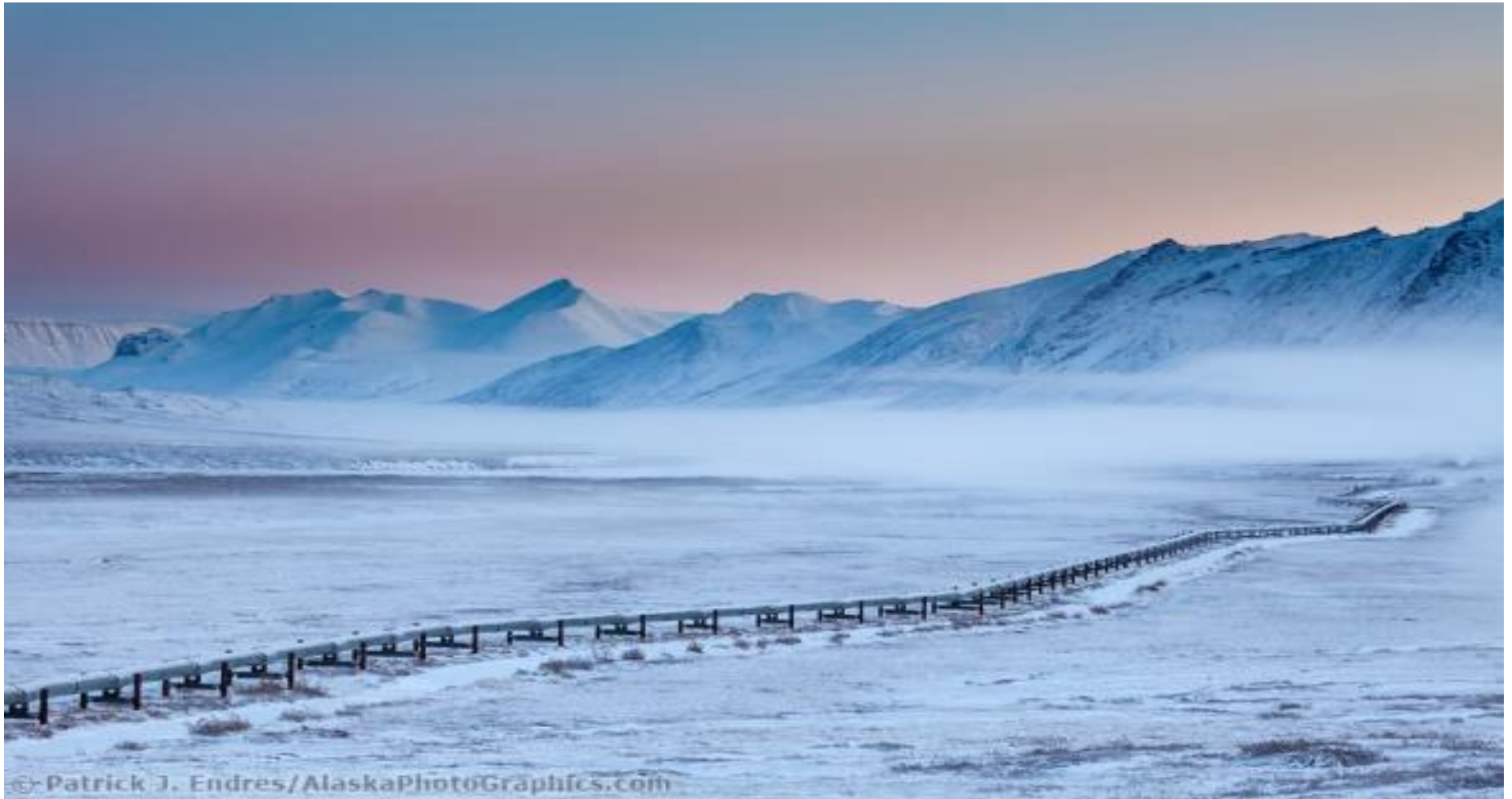
Trans Alaska oil pipeline in the north side of Antigon
