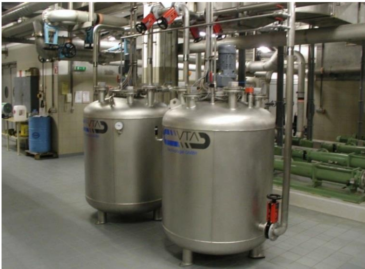
Ultrasonic plant Villach WWTP (Austria) (Designed for 100 m 3 /d sludge with 6%DS)
