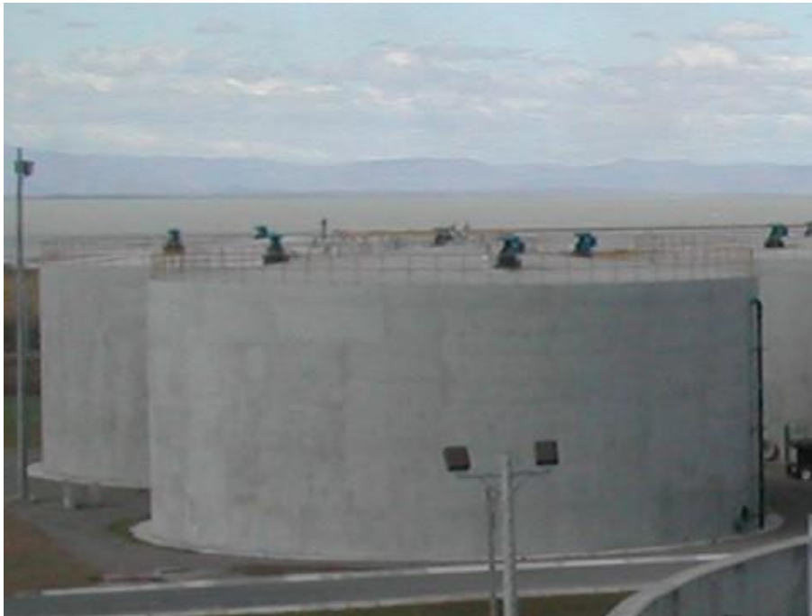
Cylinder shaped digester
