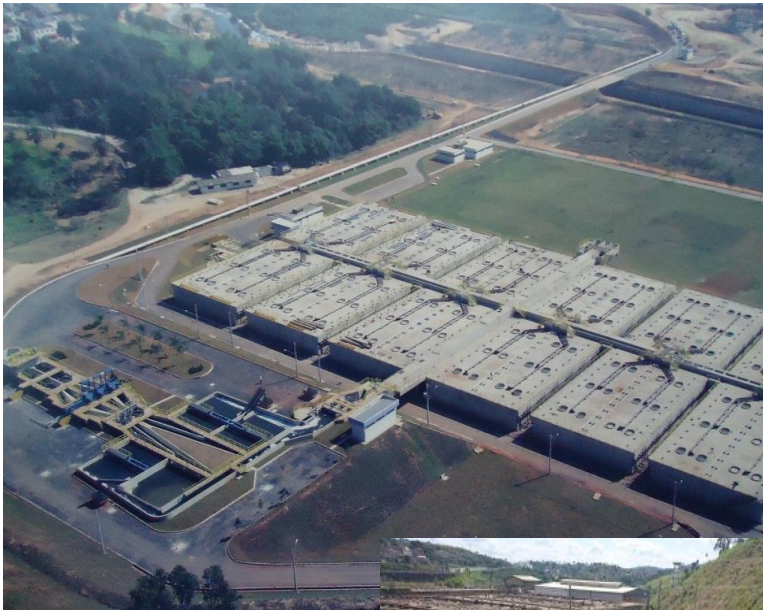
UASB technology: Onca WWTP (Brazil)
