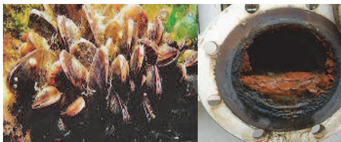
Fig. 21. Mussels development on intake (left) and biofilm on pipes (right)
