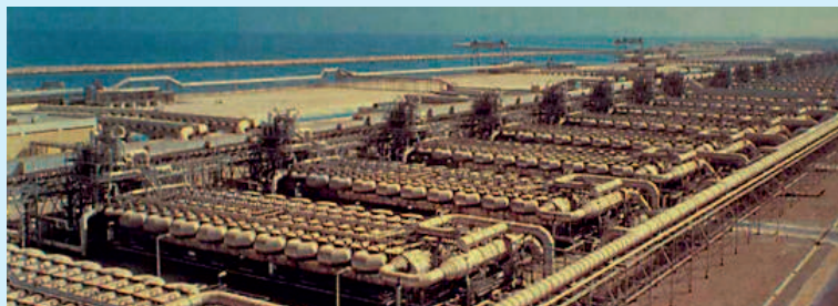
Figure 12. A few of the 40 units at Al-Jubail Phase 2, each 5 million GPD
