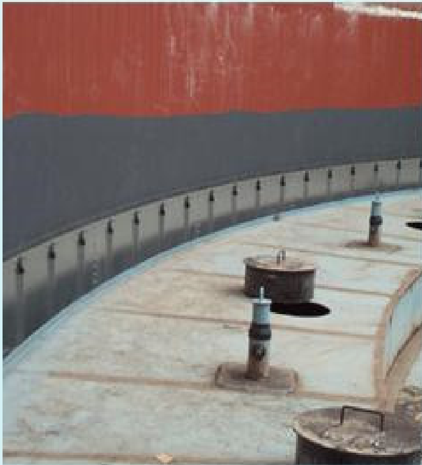
( WB-1 Pantograph Type Mechanical Shoe Seal )
