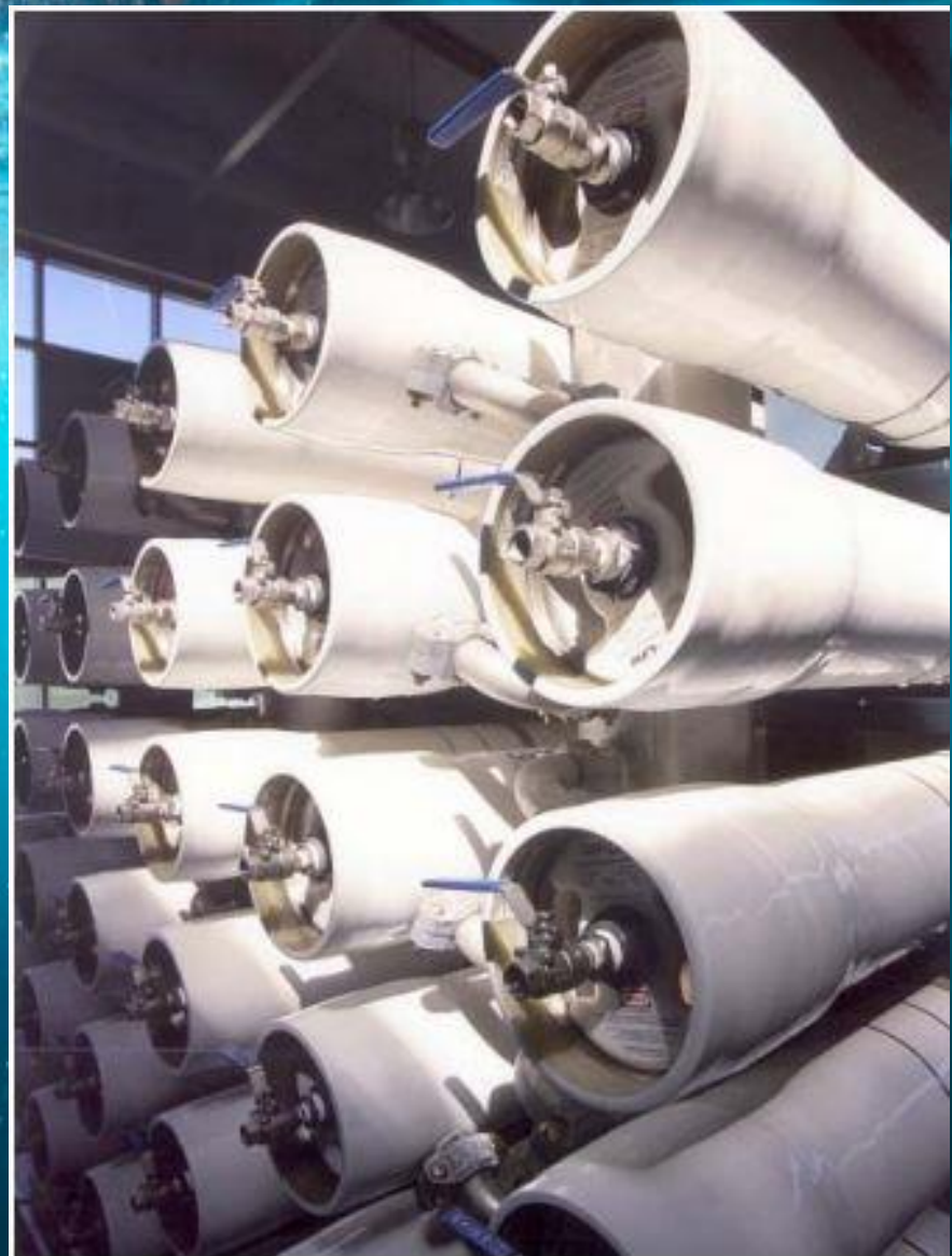
Stack of pressure vessels
