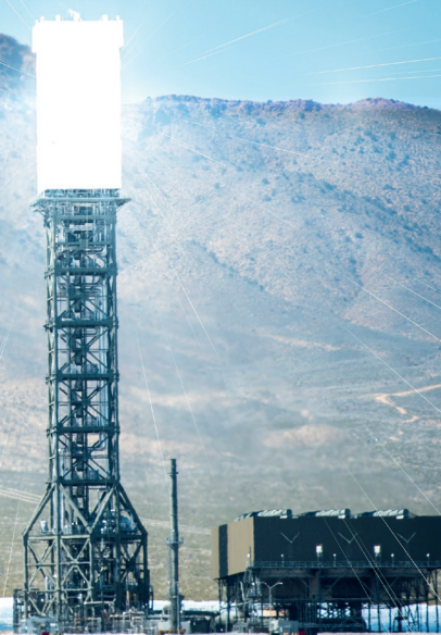
Concentrated solar power
