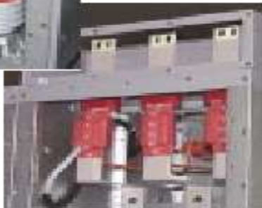
Bus risers to bus duct or roof busings
