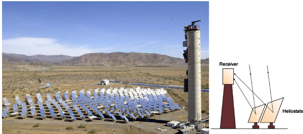
Fig. 18. Principle of a point focusing solar tower system (Plataforma Solar de Almería, Spain) [6].
