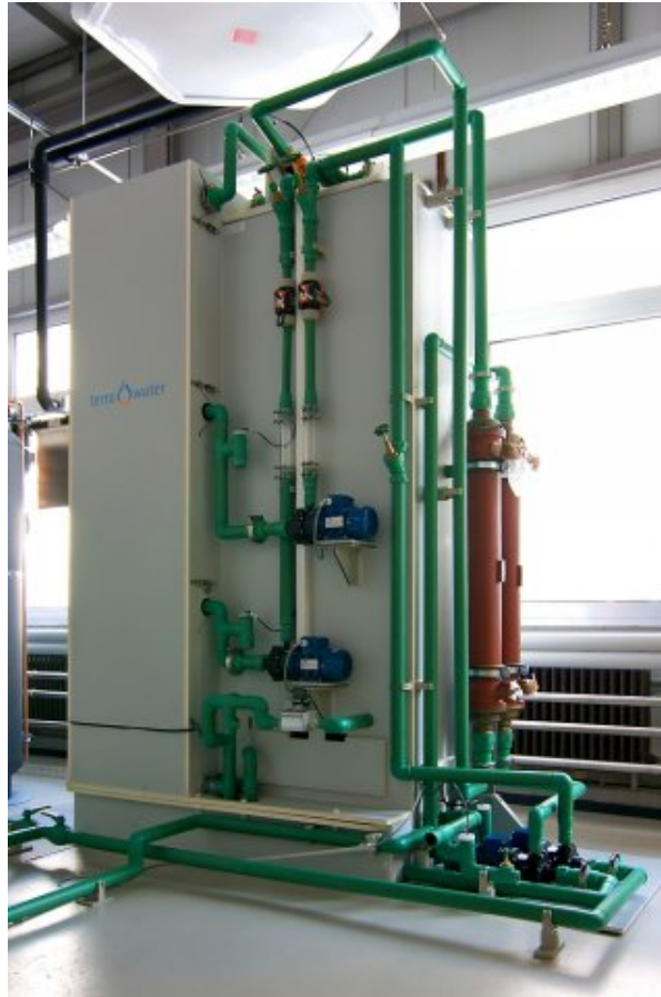
Fig. 4.4.: Water desalination from Terrawater which is used in the project in Egypt [Ter10]. The photo was taken at the company in Kiel.
