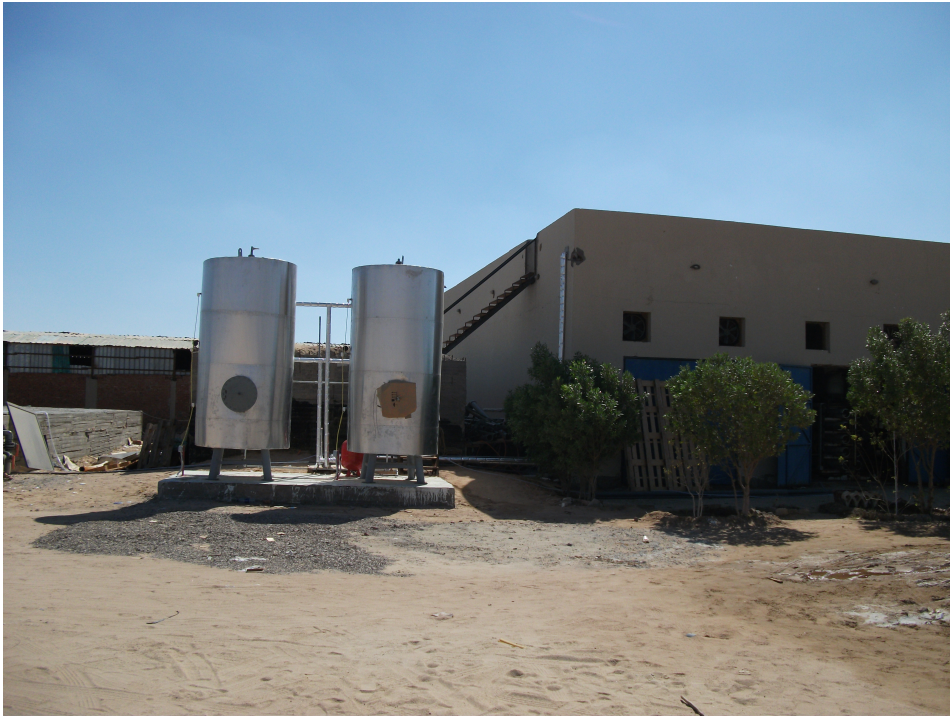
Fig. 5.9.: Building site of the demonstration plant with two Sunwater heat storage tanks.
