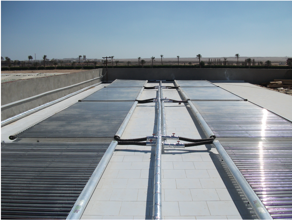
Fig. 5.10.: Installation of the vacuum tube collectors at the roof of the building. In the background at the left is the weather station.
