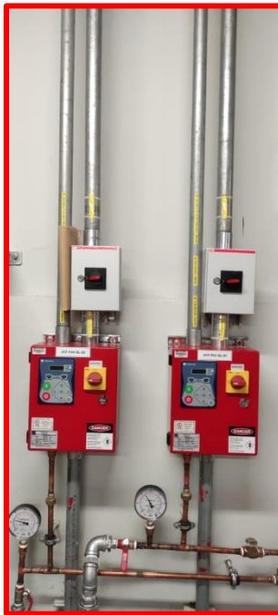
FIGURE A.4.31(a) Piping Connection for Each Automatic Pressure Switch (for Electric-Driven and Diesel Fire Pump and Jockey Pumps).
