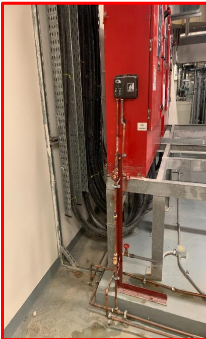
FIGURE A.4.31(a) Piping Connection for Each Automatic Pressure Switch (for Electric-Driven and Diesel Fire Pump and Jockey Pumps).
