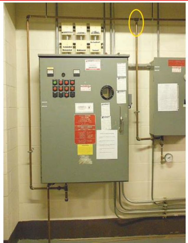
FIGURE A.4.31(b) Piping Connection for Pressure Sensing Line (Diesel Fire Pump).
