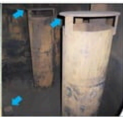
Disc Type Vortex Breakers in a Tower
