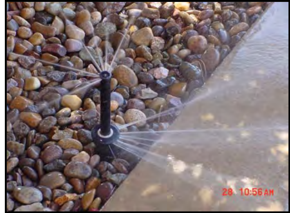
Figure 2-1: Sprinkler Leak
