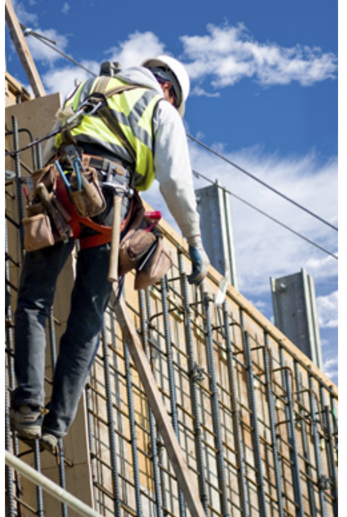
A worker using fall arrest equipment. Note the full body harness with lanyard attached at the back.
