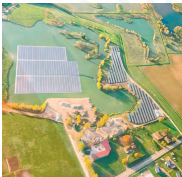
Amarenco's Floating PV site in Montpezat, France.
