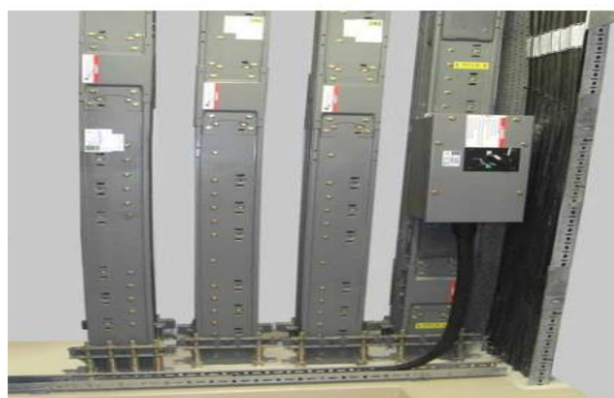
Typical busbar riser system including plug-in circuit breaker
