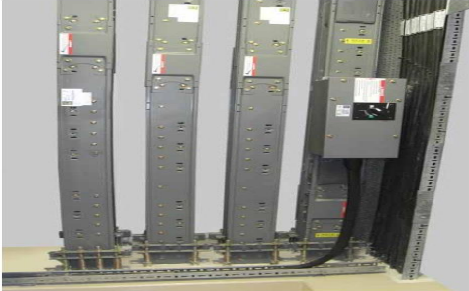
Typical busbar riser system including plug-in circuit breaker
