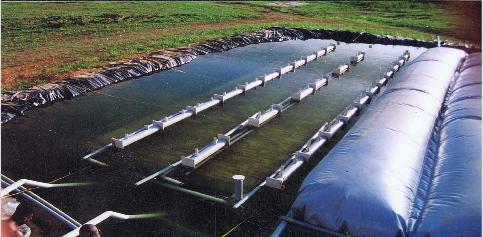
Natural UASB-Pond constructed in Jamaica
