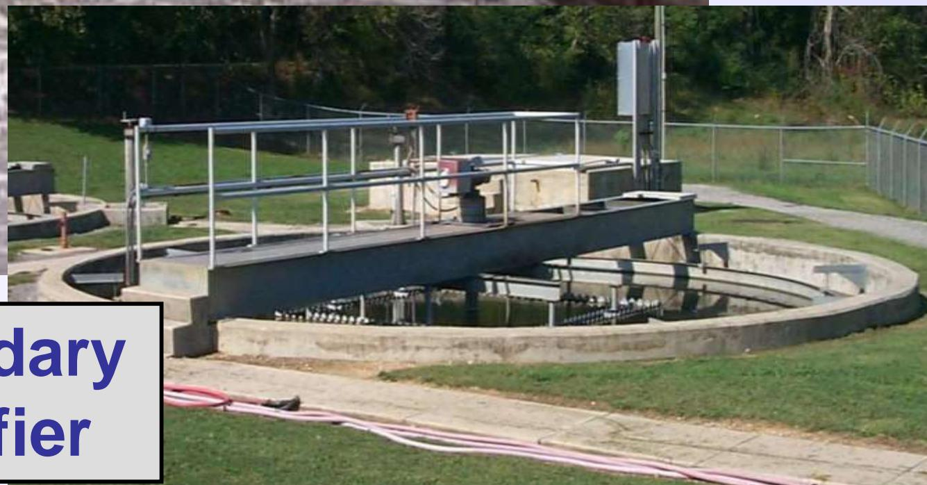
A photograph of a circular concrete secondary clarifier. The structure is surrounded by a metal walkway with railings. The water inside the tank is clear. In the foreground, a red and white striped hose lies on the grass. The background shows a grassy area and a fence.
