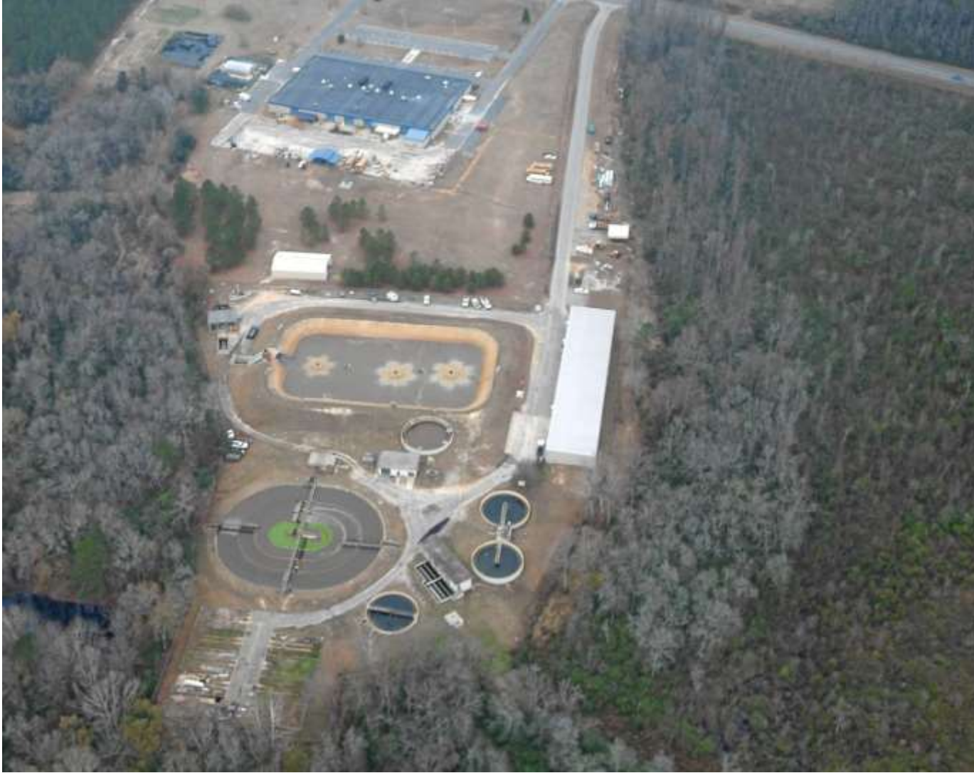
5 MGD Dillon Wastewater Treatment Plant Dillon, South Carolina USA
