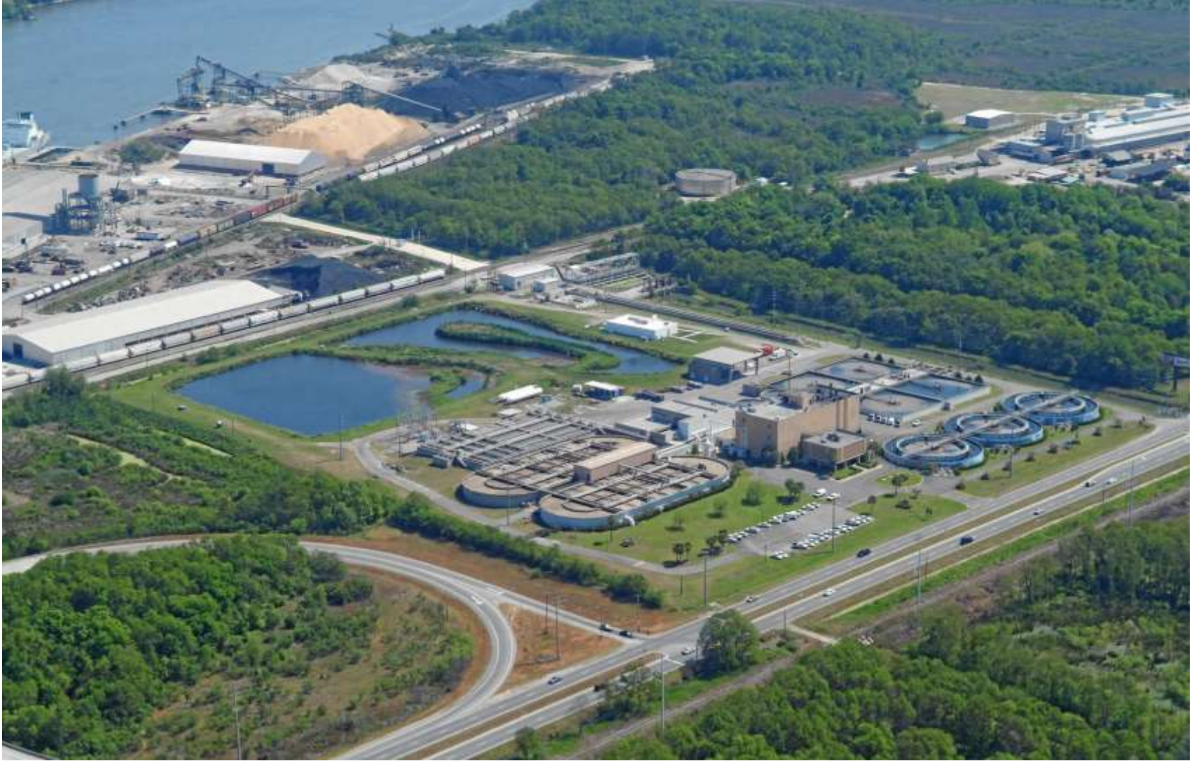
President Street Wastewater Treatment Facility Savannah, Georgia USA
