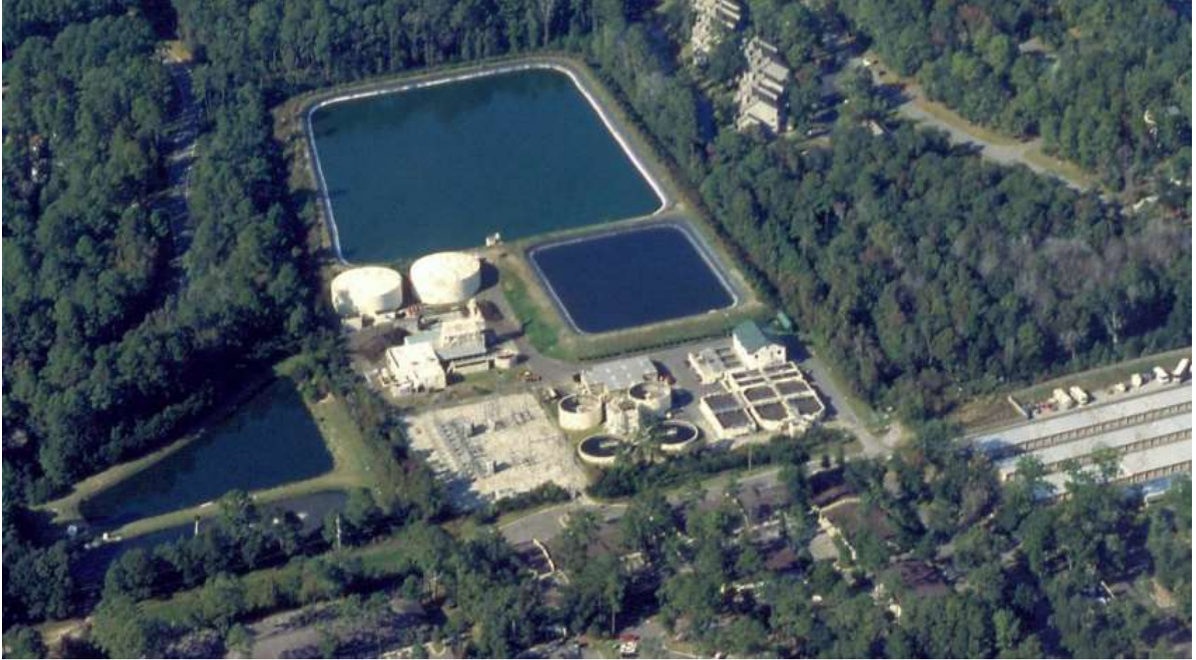
2.1 MGD Wastewater Treatment Plant - Broad Creek Public Service District Hilton Head Island, South Carolina USA
