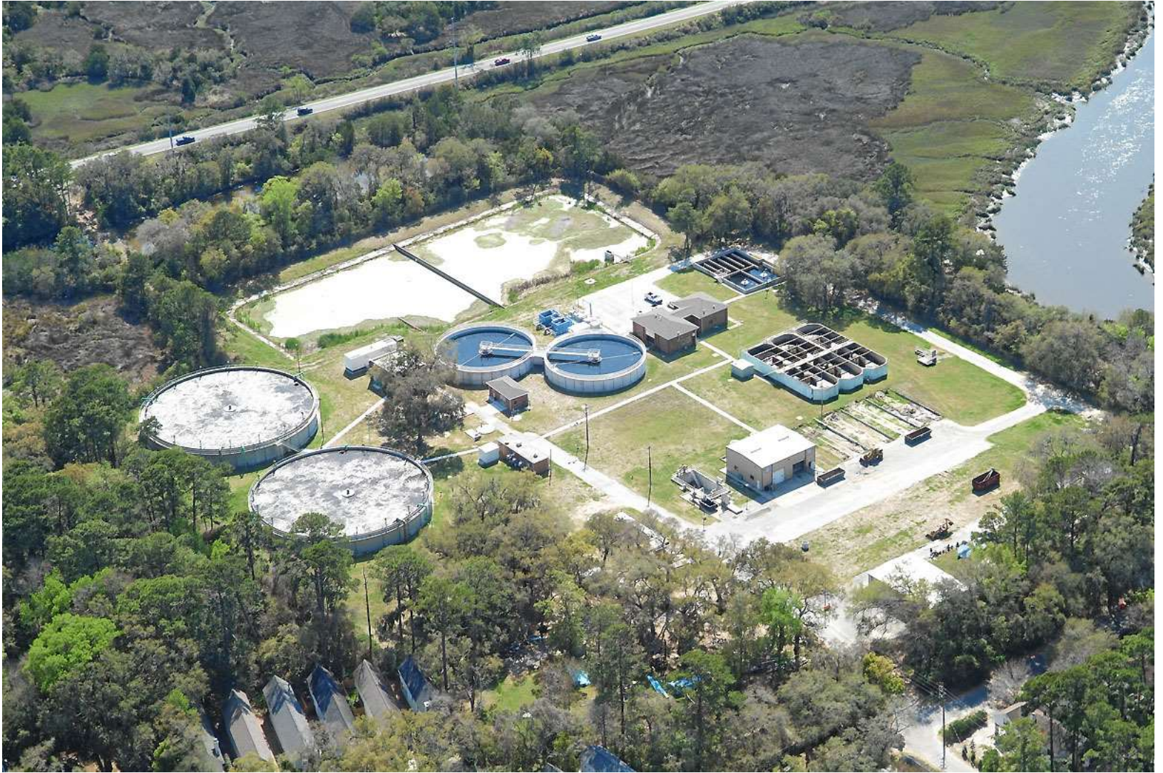
4 MGD Wastewater Treatment Plant St. Simon's Island, Georgia USA
