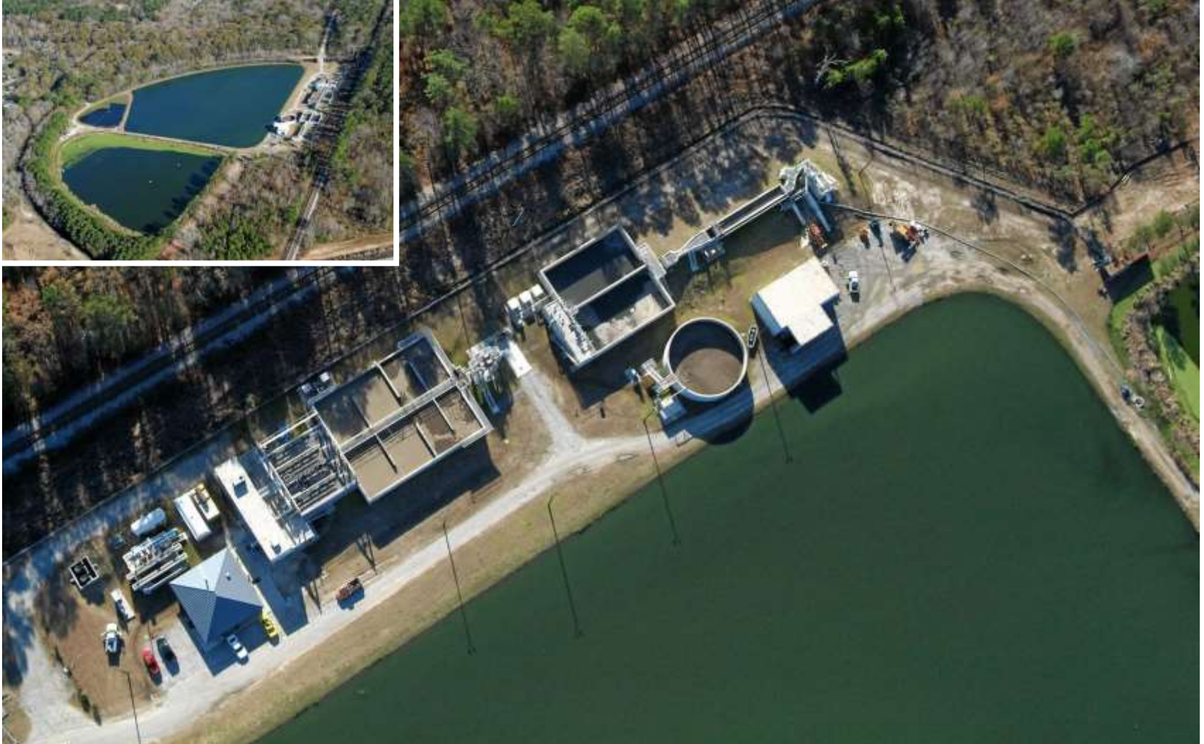
2.5 MGD Wastewater Treatment Plant Membrane BioReactor Pooler, Georgia USA
