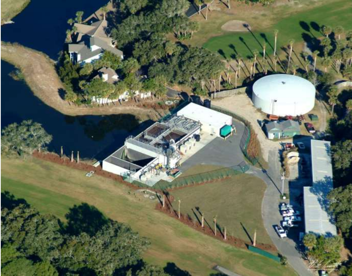
0.67 MGD Fripp Island Wastewater Treatment Plant Fripp Island, South Carolina USA
