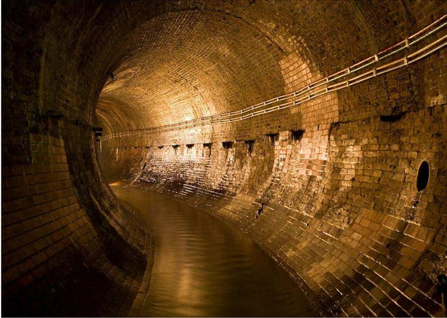
Brickwork sewer line
