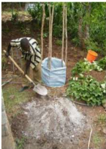
Construction of a Greywater Tower in Arba Minch Town, Ethiopia. Source: SHEWA (2009)
