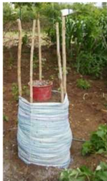
Construction of a Greywater Tower in Arba Minch Town, Ethiopia. Source: SHEWA (2009)
