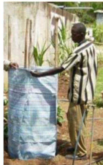
Construction of a Greywater Tower in Arba Minch Town, Ethiopia. Source: SHEWA (2009)
