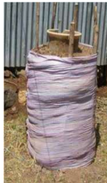
Construction of a Greywater Tower in Arba Minch Town, Ethiopia. Source: SHEWA (2009)
