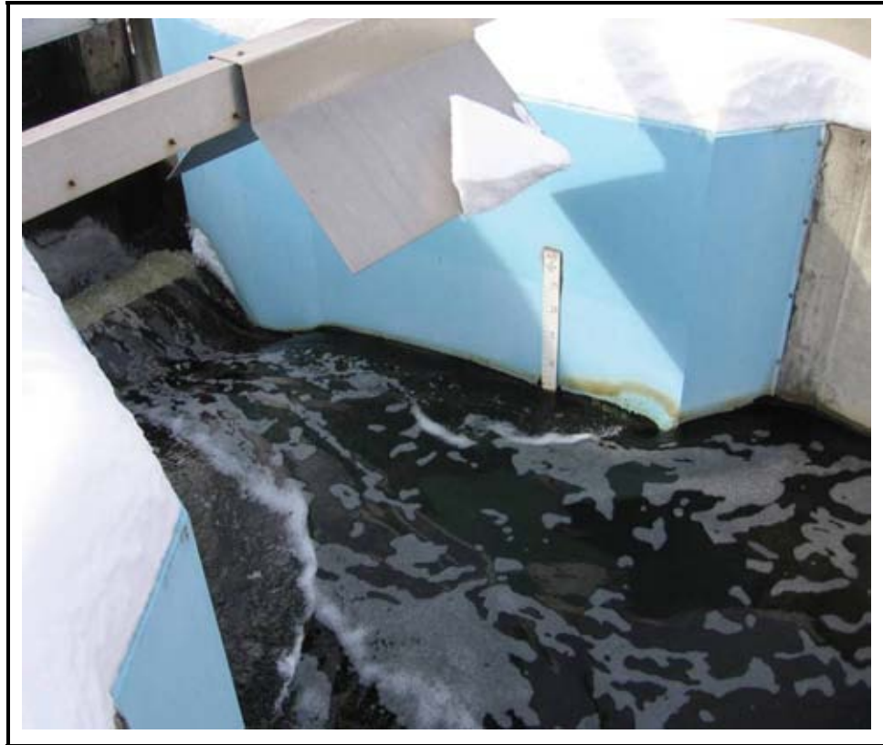
Figure 9-2 - Example Installation of a Parshall Flume with a Staff Gauge at Secondary Device Location
