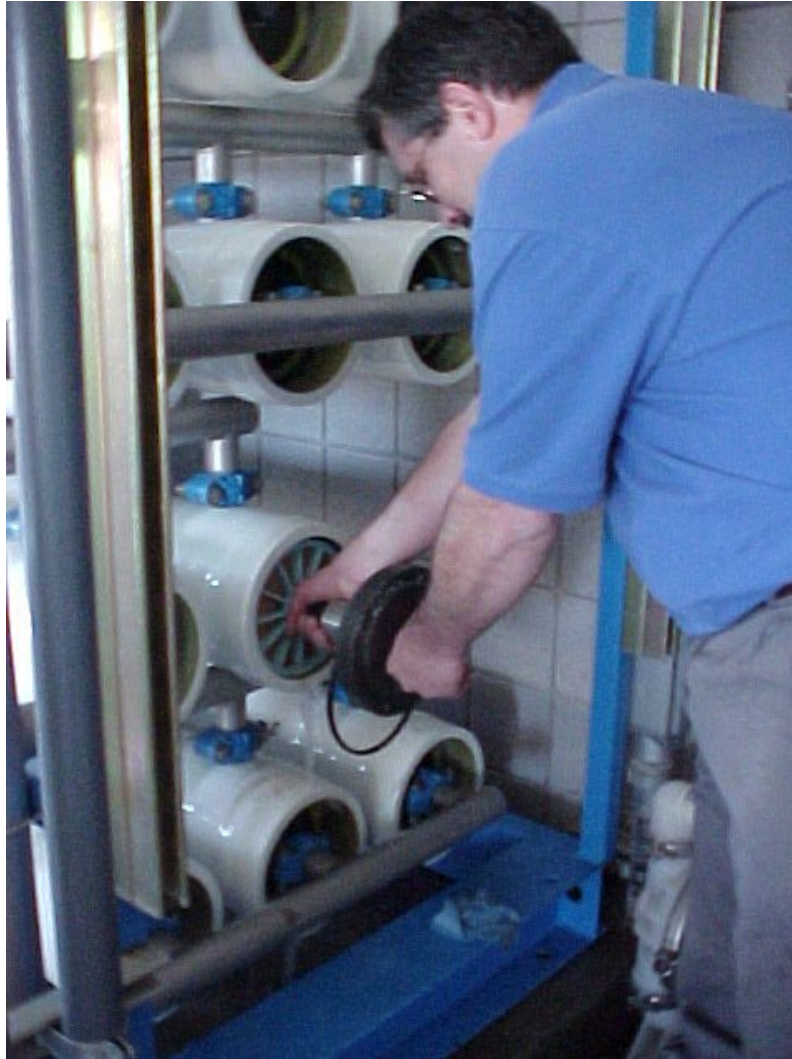
Changing the membrane filter on a RO unit.
