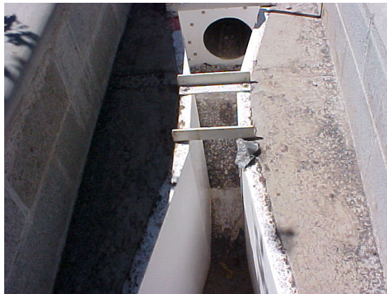
Parshall Fume and Ultrasonic Flow Meter Notice the debris and most POTW's will write a NOV for uncleanness.
