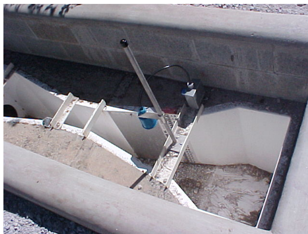
Parshall Fume and Ultrasonic Flow Meter Notice the debris and most POTW's will write a NOV for uncleanness.
