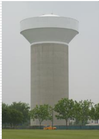
Water tank pressure
