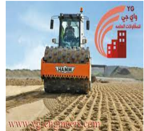
Soil Compaction
