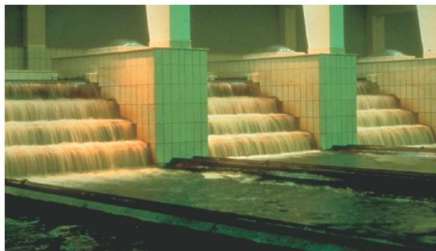
Figure 7 - Treatment of slightly anaerobic groundwater
