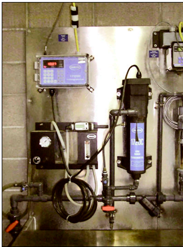
Figure 2-2 On-line sampling and monitoring equipment
