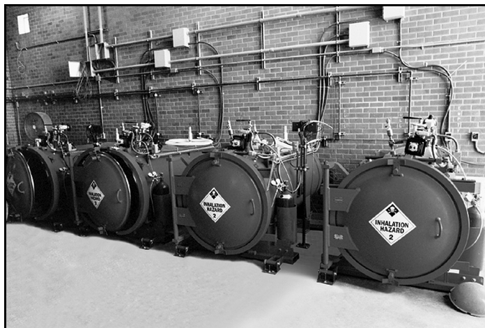
Figure 4-19 Example of total cylinder containment
