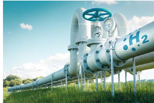
Pipeline Delivery Long Distance
