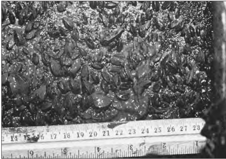
Figure 9-3 Zebra mussels encrusted on structure
