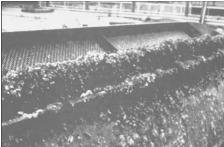
Figure 9-5 Impact of zebra mussels on screens
