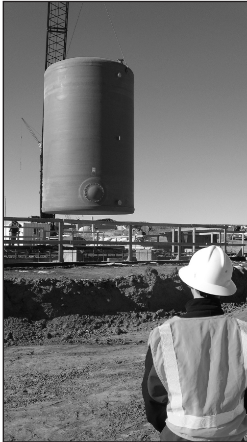
Figure 4-2 Installation of water tank (courtesy Aurora Water)
