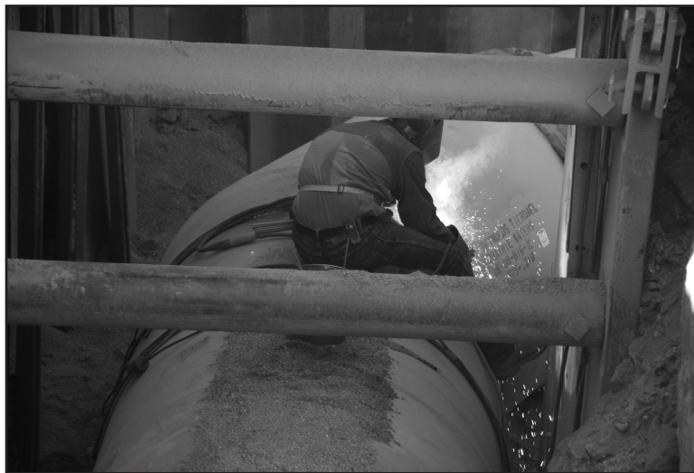
Figure 3-3 Pipeline repair
