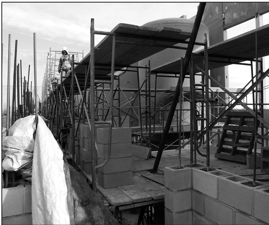
Figure 4-1 Contractors following safety procedures (courtesy Aurora Water)
