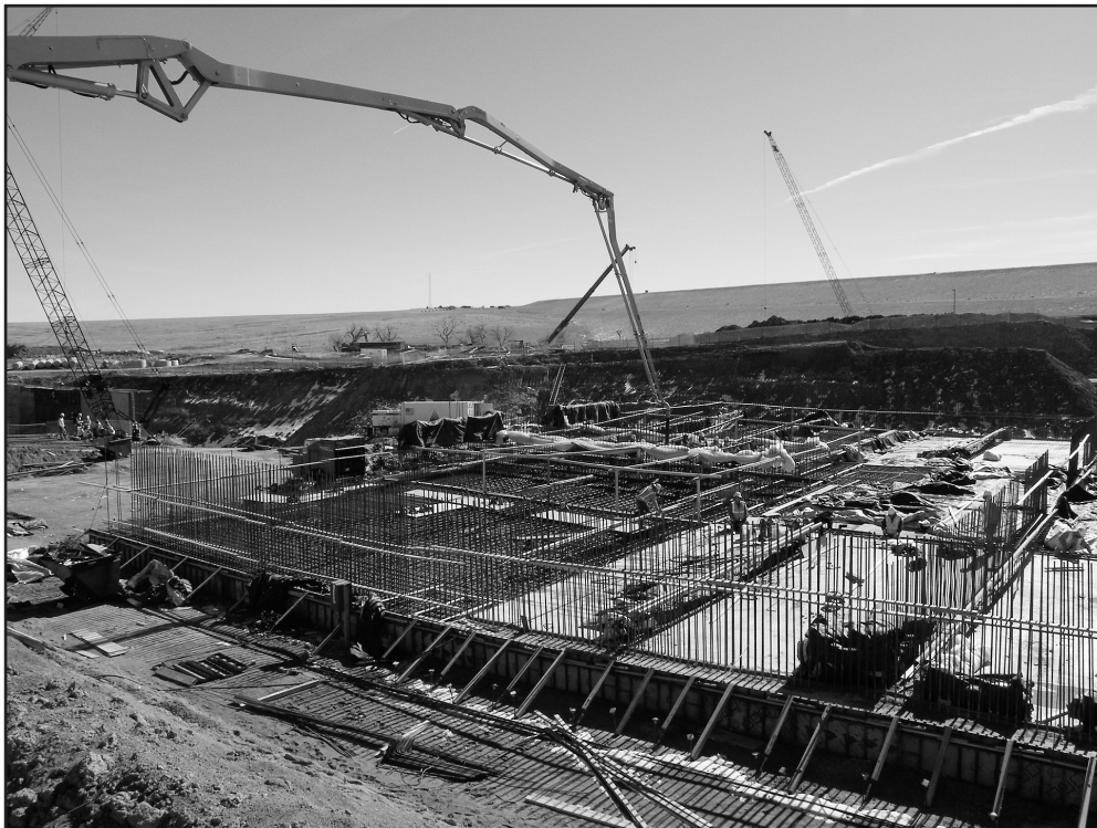
Figure 4-3 Workers involved in plant expansion (courtesy Aurora Water)
