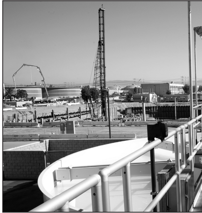
Figure 8-3 Site and foundation work
