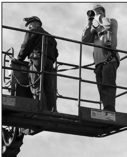
Figure 11-2 Documentation of equipment installation procedure
