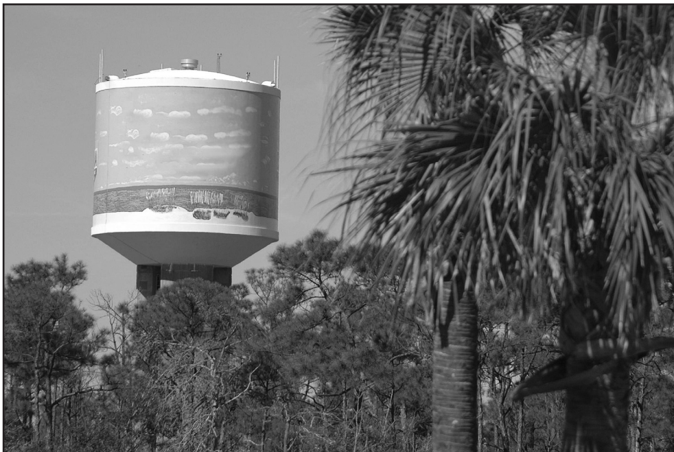
Figure 7-1 Elevated steel reservoir
