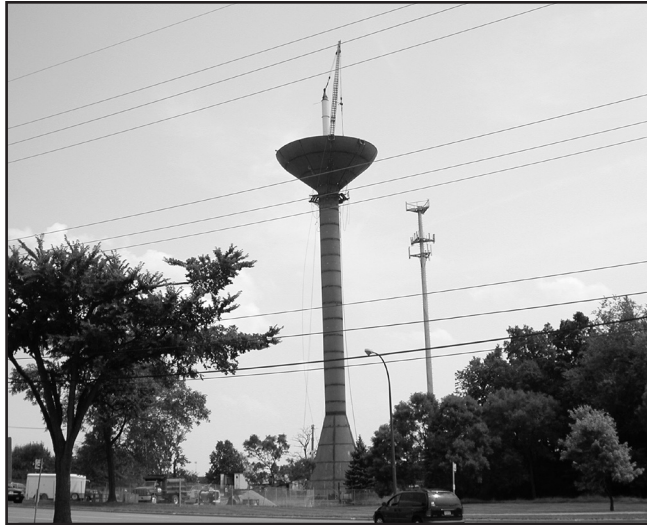
Figure I-2 Steel water tower (courtesy of B. Steglitz)
