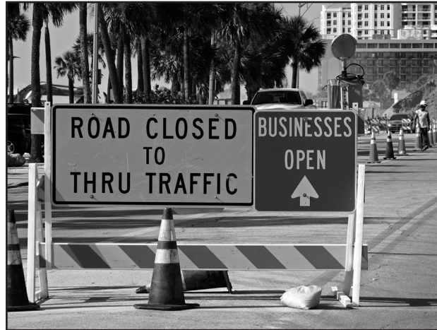
Figure 14-2 Construction signage displaying a concise message
