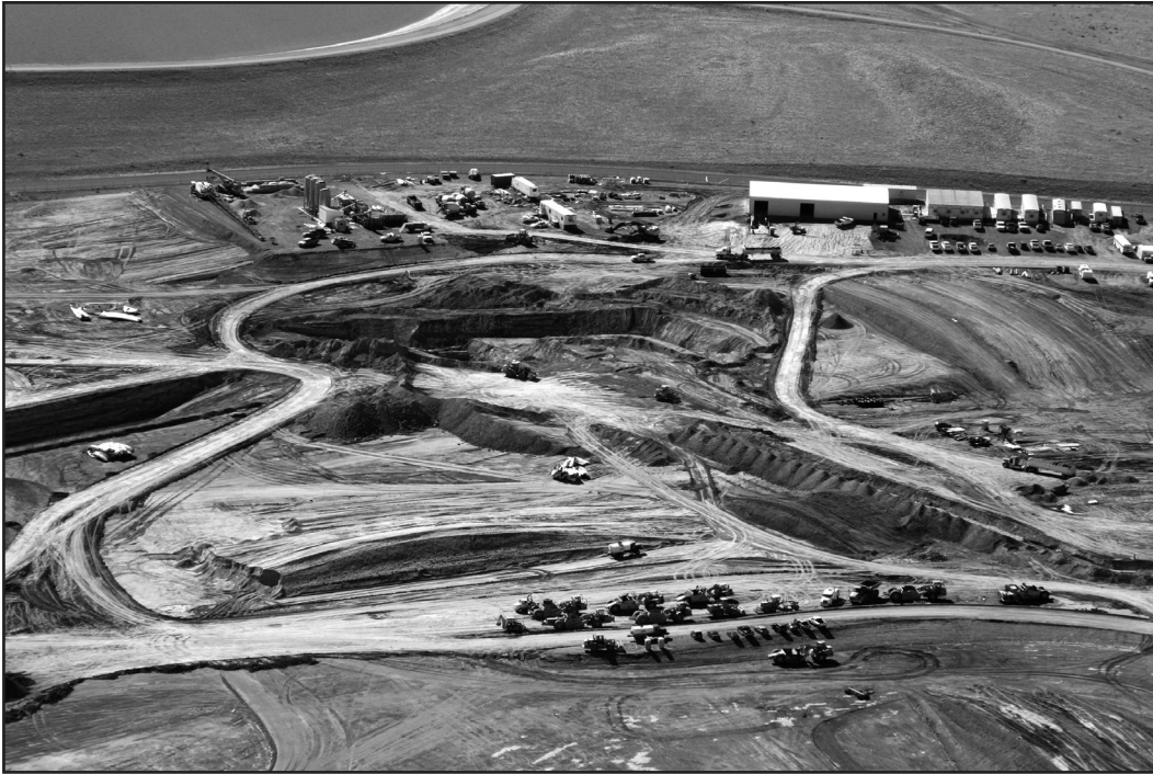
Figure 6-3 Preliminary site work (courtesy Aurora Water)
