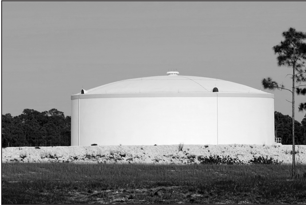
Figure 7-2 Ground storage reservoir
