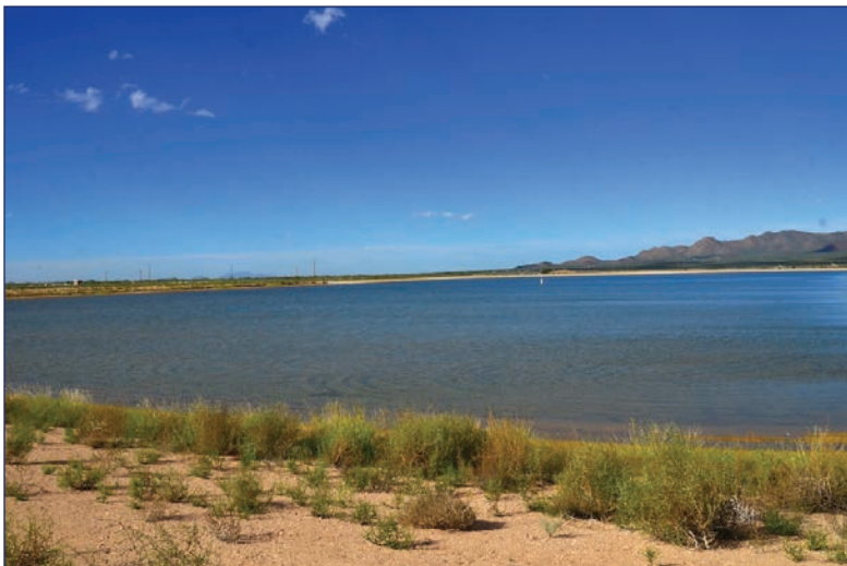
FIGURE 4.7 One of several groundwater recharge basins of the Southern Avra Valley Storage and Recovery Project (SAVSARP) used to recharge the aquifer with Colorado River water.
