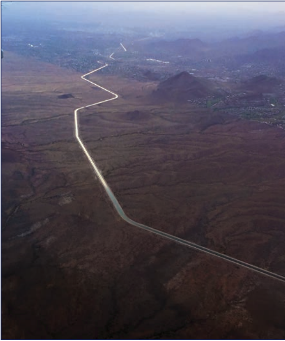
FIGURE 2.3 Central Arizona Project—CAP—canal.
