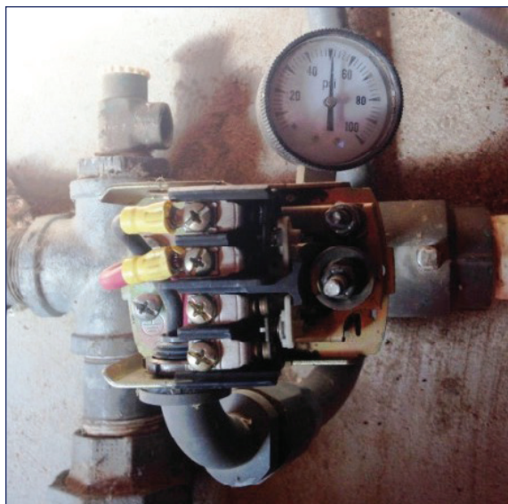
FIGURE 5.8 Captive air bladder tank pressure switch.
