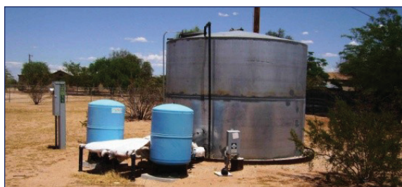
FIGURE 5.9 A shared well system with above ground storage and two pressure tanks, delivering water to two households.
