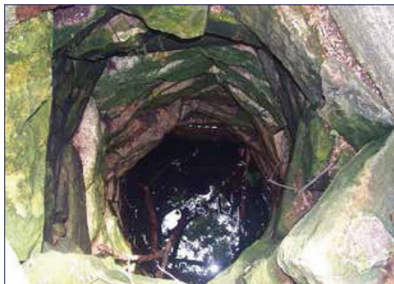
FIGURE 10.4 Unplugged, abandoned wells can be a source of groundwater pollution and maybe a safety concern.
