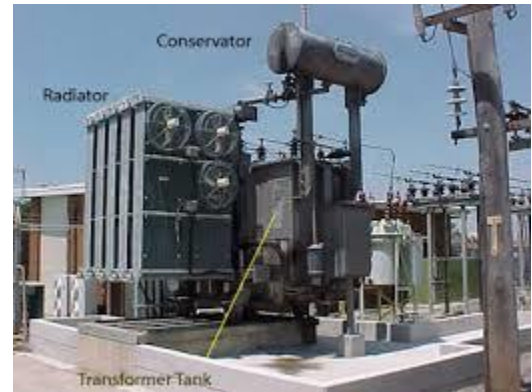
Figure 190: Conservator installation
