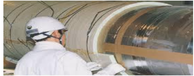
Figure 131: insulation material installation and securing
