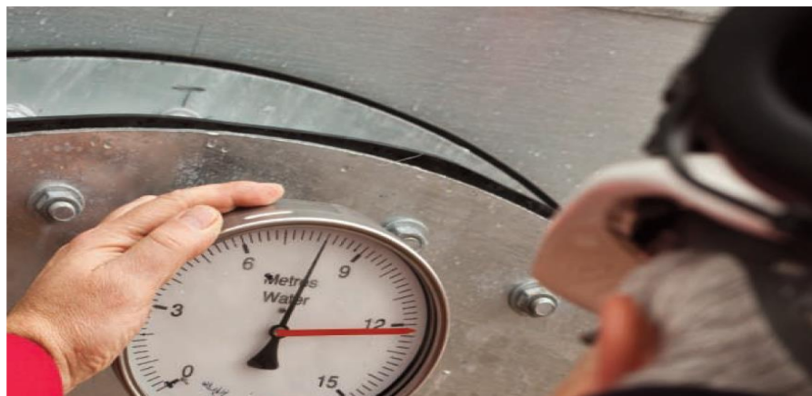
Figure 70: Testing and commissioning
