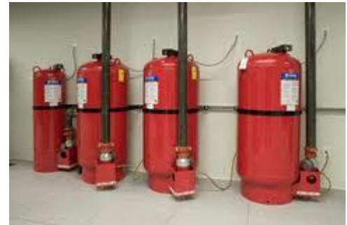
Figure 58: cylinder positioning
