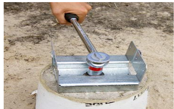
Figure 156: anchor bolt tightening
