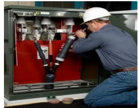
Figure 196: Termination
