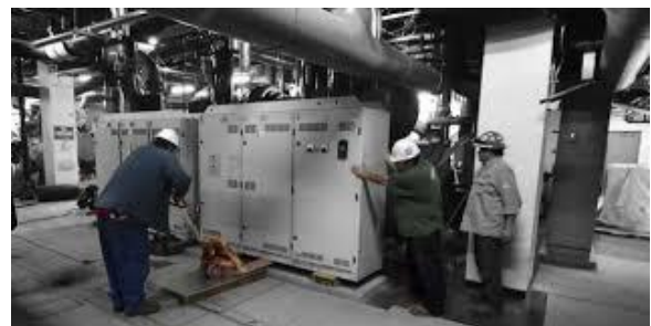
Figure 185: Securing to foundation
