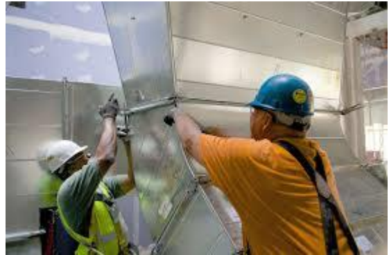
Figure 138: Duct installation
