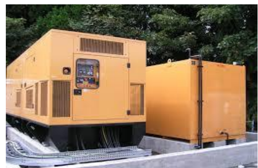
Figure 125: Fuel tank installation
