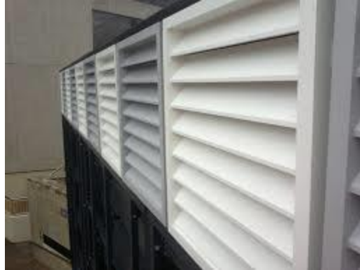
Figure 153: Louvre installation
