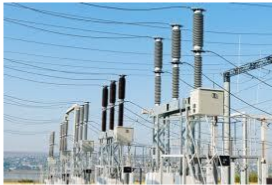
Figure 178: Electrical supply commission
