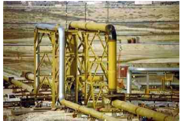
(b) Fabricated Expansion Loops
