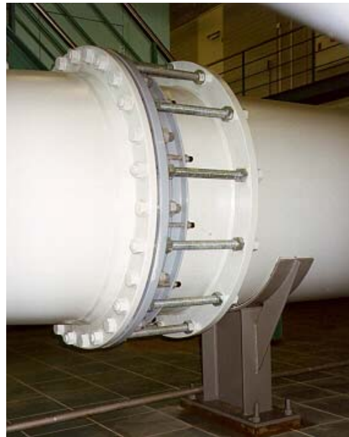
(b) Two Designs of Pipe-to-flange Adapters Fitted
