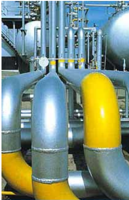
Figure 3.7: Butt-welded Joints
