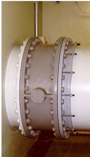
(b) Two Designs of Pipe-to-flange Adapters Fitted
