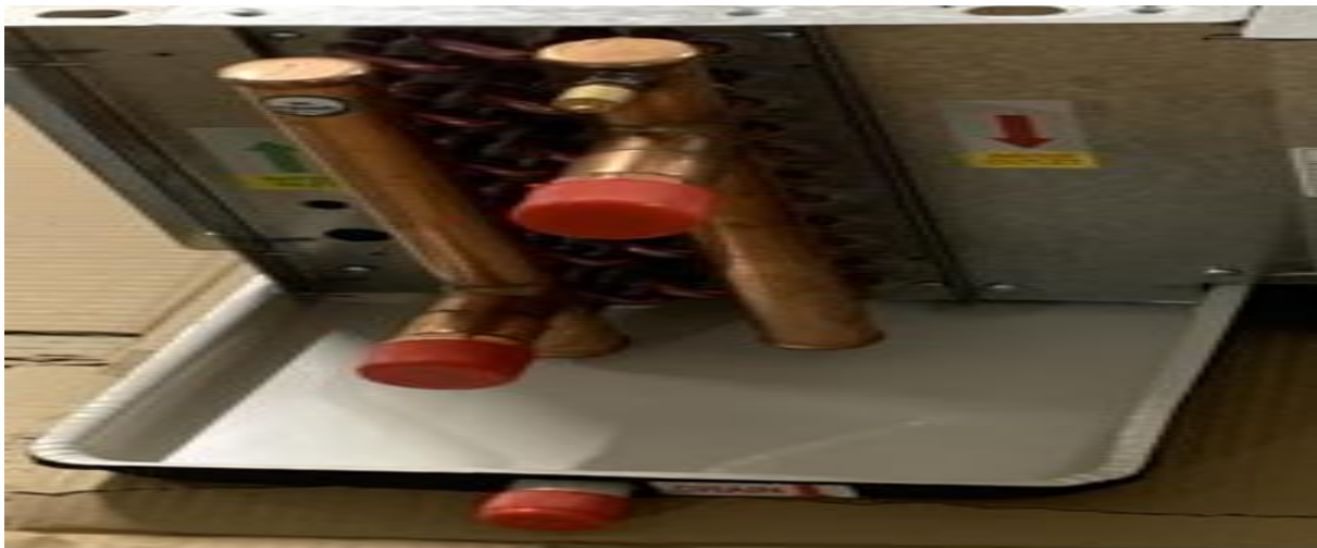
FCU Condensate Drain Pan
