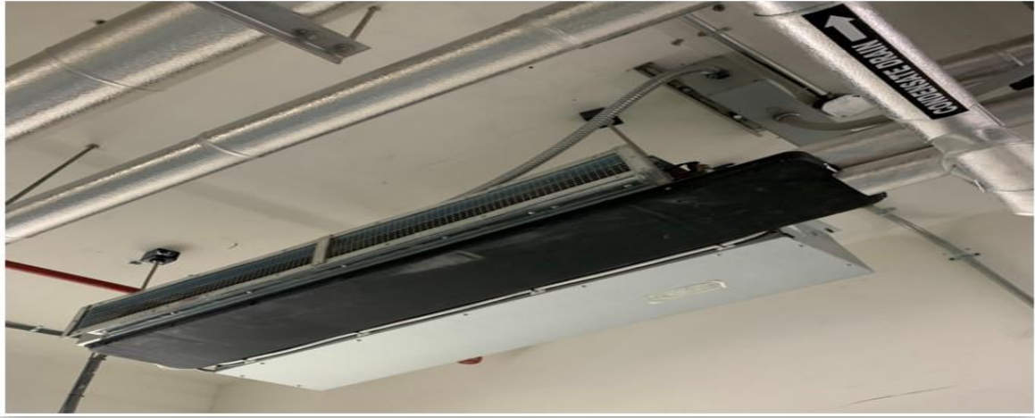
FCU Install exposed at mechanical room
