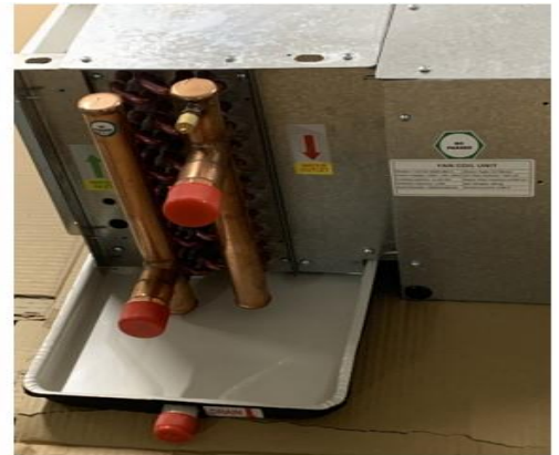
FCU with Cooling Coil and Electrical Heater
