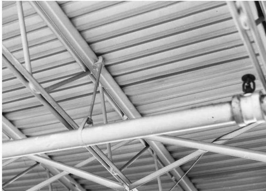
Photo 8 A hanger assembly consisting of a top-beam clamp, 3/8" threaded rod, and a standard swivel ring.
