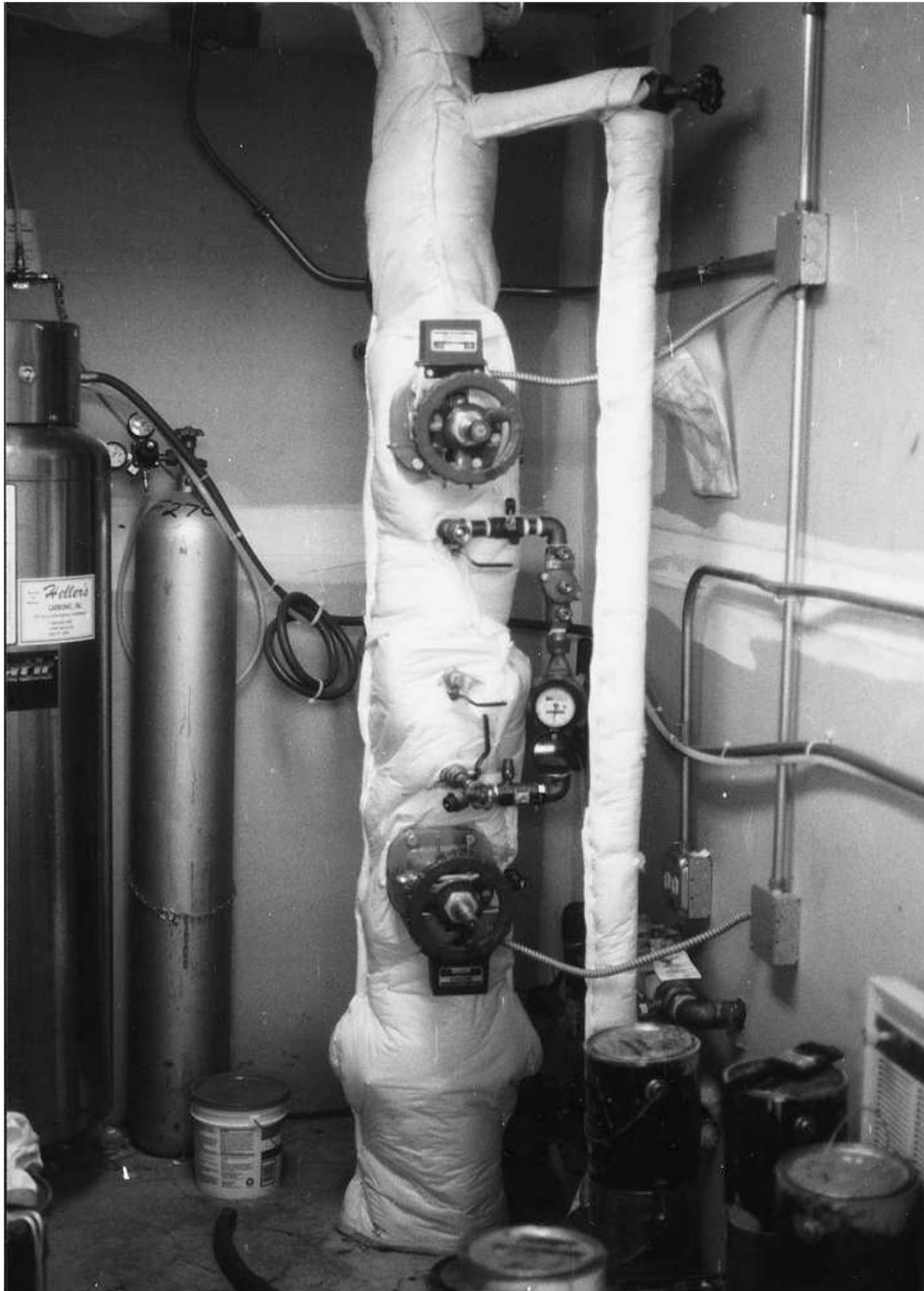
Photo 4 This is the resulting installation from the plan drawing depicted in Figure L-15. The fire department connection has been moved during installation to a different location. As a precaution against freezing, the contractor installed pipe covering around all piping including the main drain line, with the exception of the valve stems, pressure gauge, and the metered backflow preventer by-pass. Of course, the drain piping downstream of the drain valve is dry, and some pipe covering will have to be removed if and when the backflow preventer interior requires cleaning.
