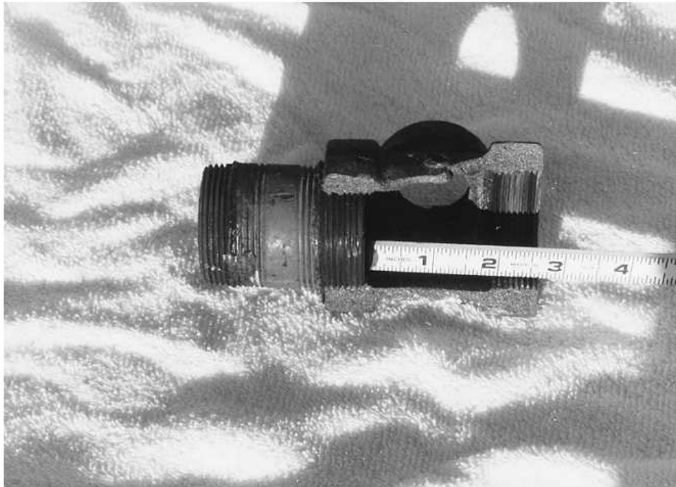
Photo 1 The end of the carpenter's rule is flush to the end of the 1 1/2" nipple. This illustrates the 1" take-out, measured on the interior of the broken fitting, of a 1 1/2" x 1 1/2" x 1" cast-iron tee.
