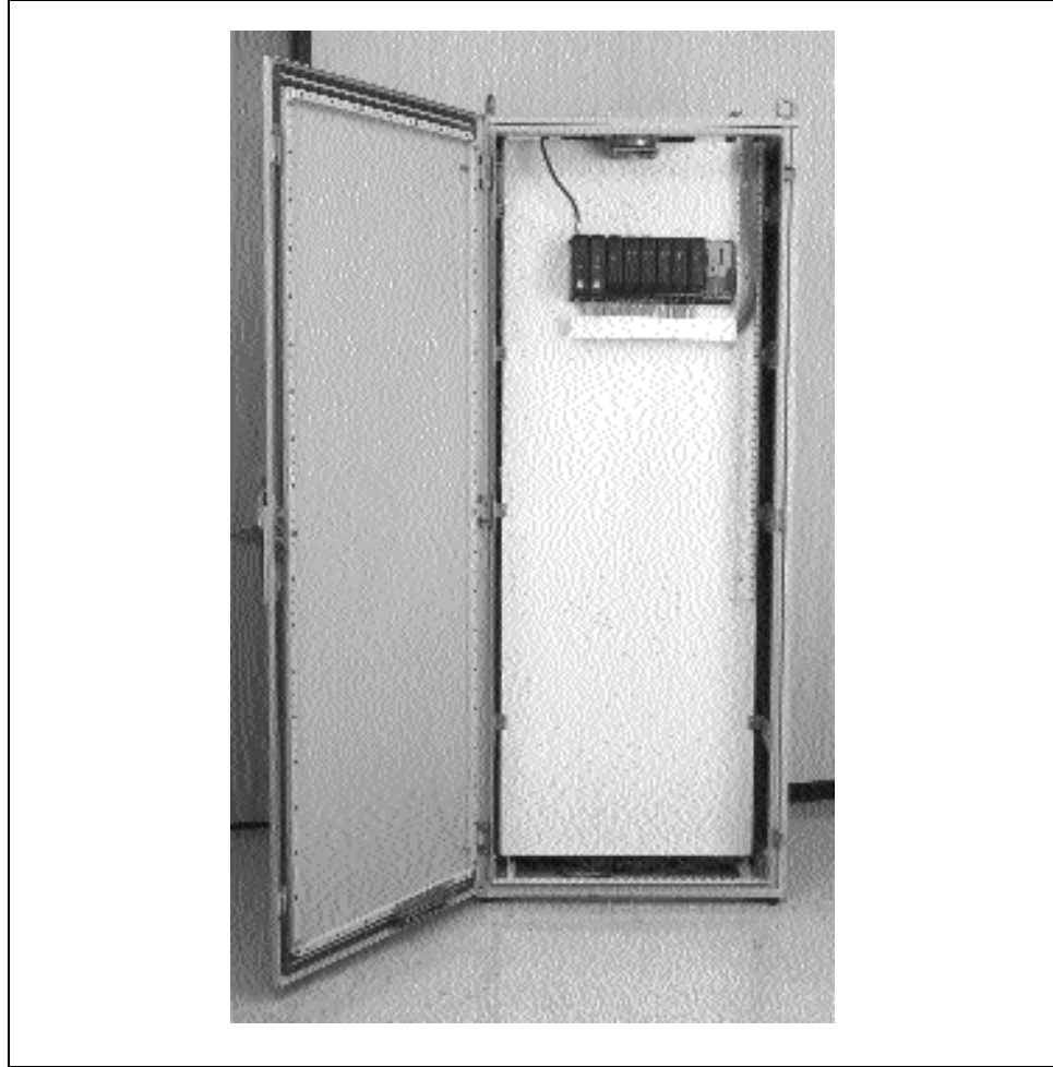
Figure 8-7b. Cabinet Footprint Using Foundation Fieldbus (Courtesy of Emerson Process Management)
