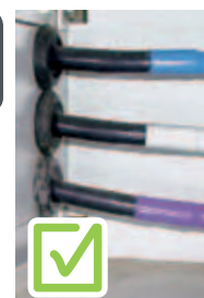
A plastic ring is used to protect cables from the hole in the sheet.
