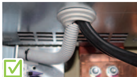
Cable glands are used to protect cables from the hole in the sheet.
