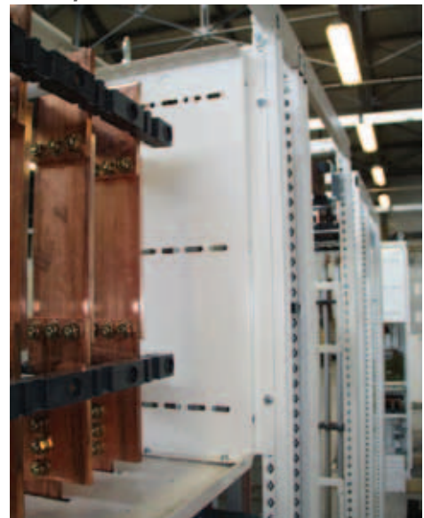
Dismountable vertical connections
