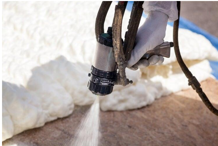
Figure 5 Illustration for spray foam insulation
