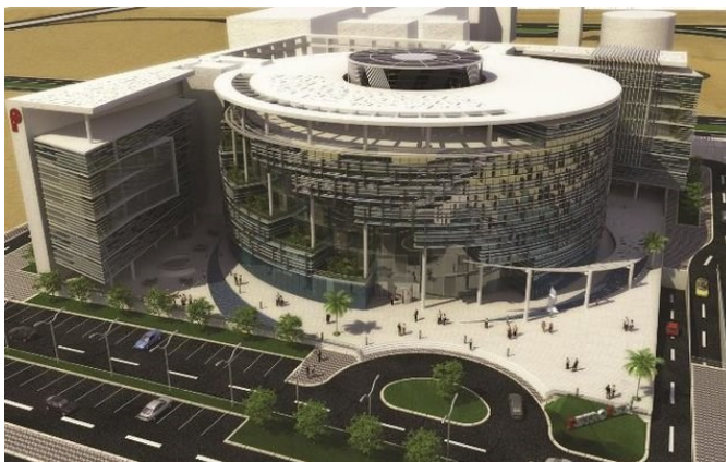
Figure 2: Petro-jet Company new head administrative office building
