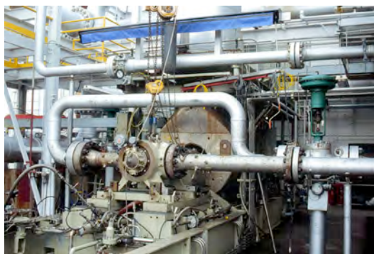
Figure 5.6 Closed-loop test facility
