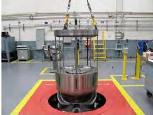
Figure 6.8 Stage 1 diffuser installation
