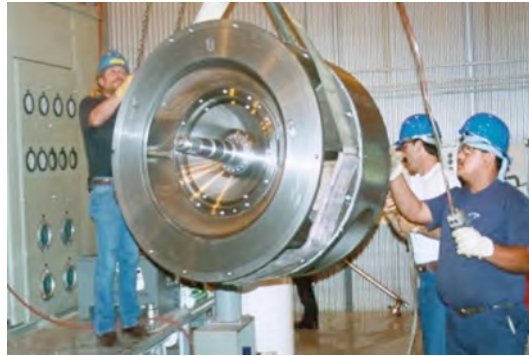
Figure 6.14 C40P module being removed for restage
