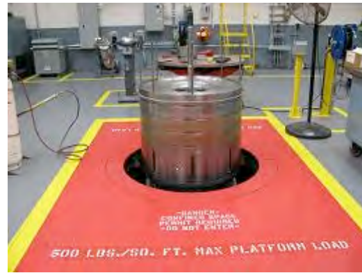
Figure 6.9 Stage 4 diffuser installed
