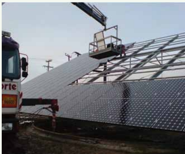
Figure 23: Module Installation on a Large Tracking System
