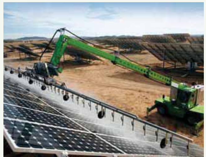
Figure 24: Module Cleaning Using Crane
