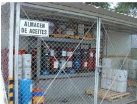
Separate and ventilated storage area for chemicals
