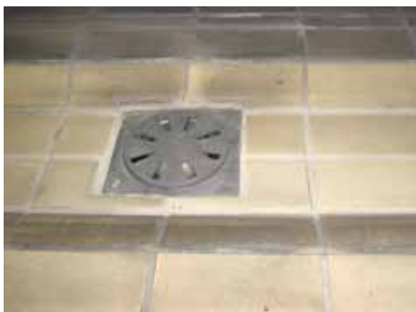
Drainage system to avoid water accumulation on the floors
