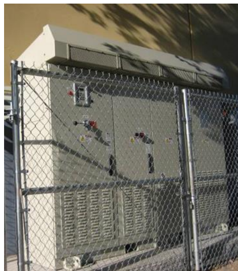
Figure 34: Central Inverters Are Used in Medium to Large Commercial Installations
