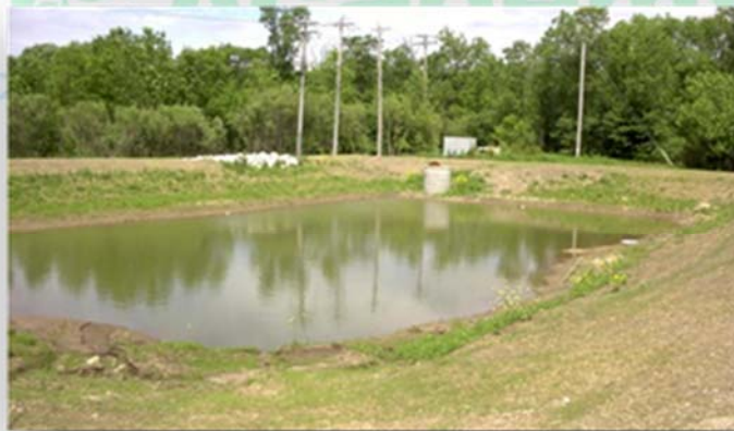
Fig 4.4 A Sediment basin in a construction site
