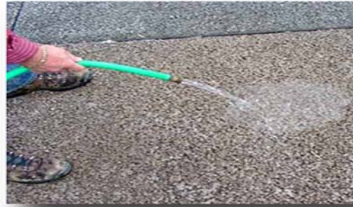
Fig 4.10 An indicative example of pervious paving
