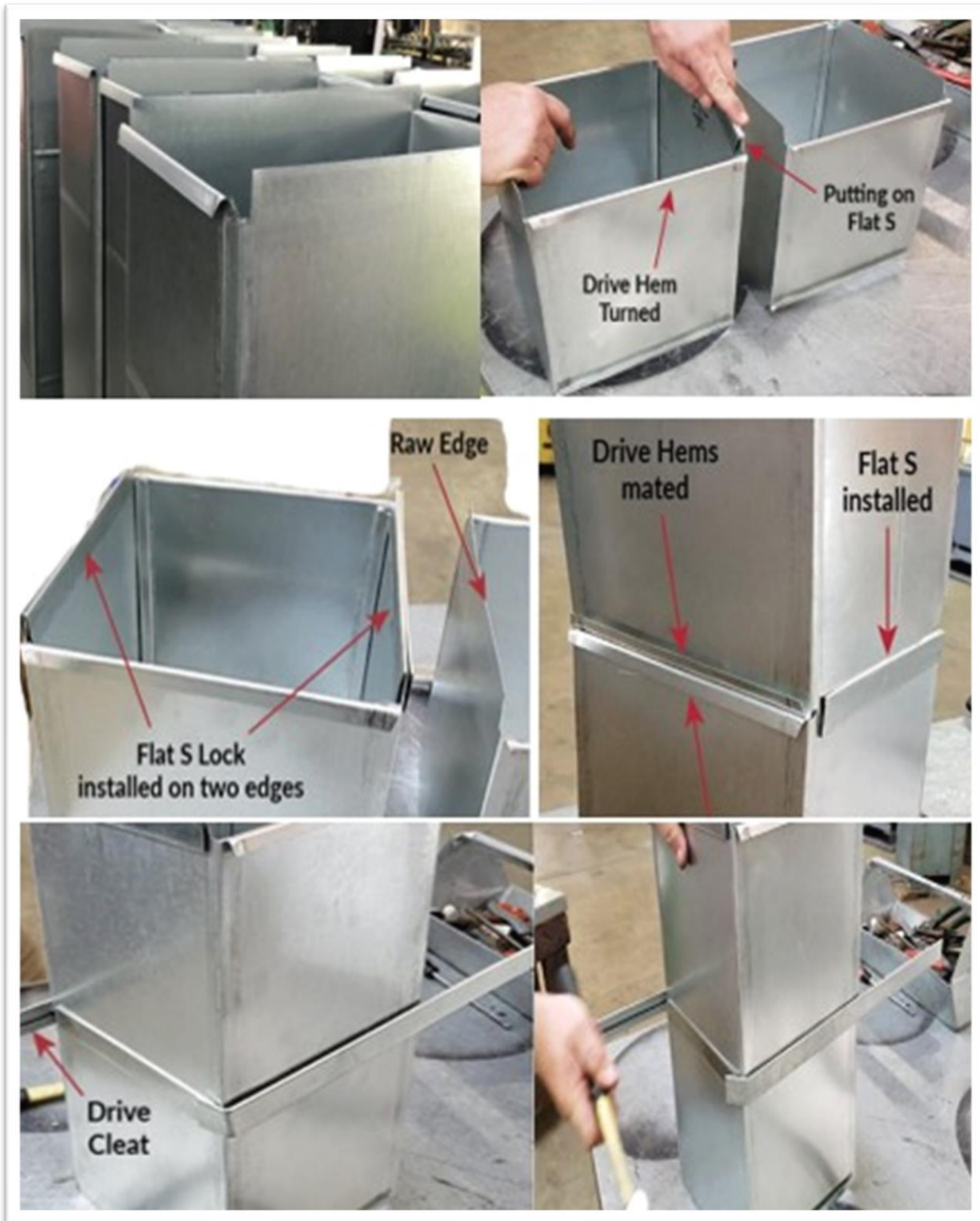
Slip and Drive Ducting Connection method
