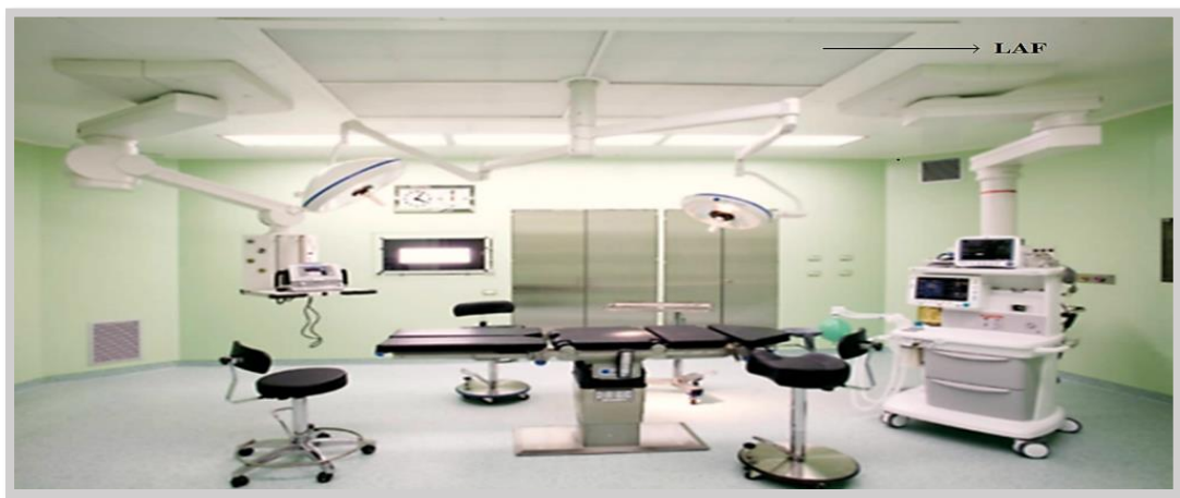
Figure 6-2 : Laminar air flow (LAF)
