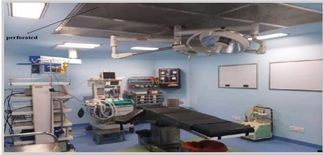
Figure 6-4 : Perforated ceiling diffuser
