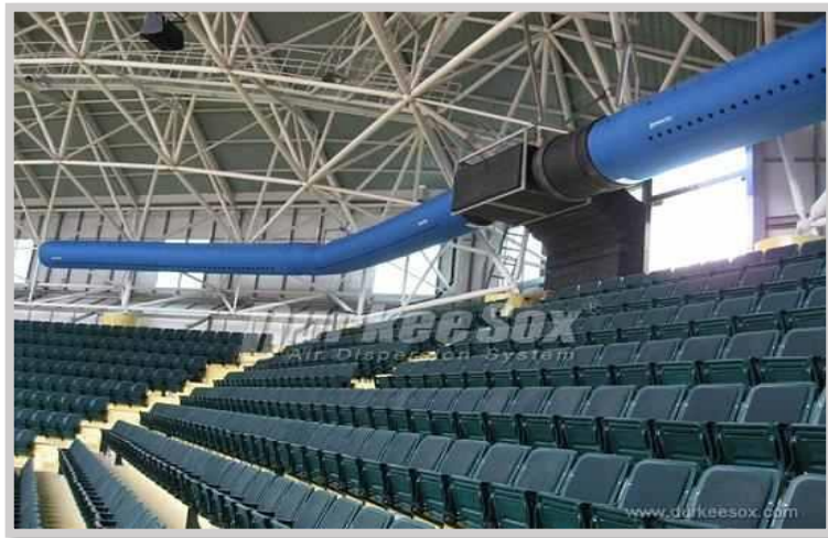
Figure 7-2 : Fabric ducts
