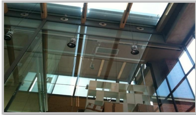
Figure 5-6 : Jet diffuser
