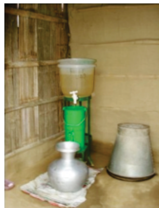
Figure 14: Read-F Arsenic Removal Unit
