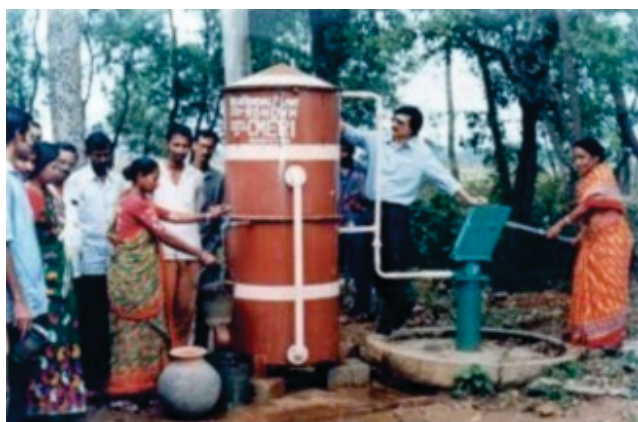
Figure 56: CMERI Iron Removal Plant
