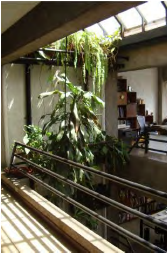
Figure 12- Transition spaces protect the air-conditioned zones and reduce the cooling demand, offer natural lighting and provide space for vegetation
