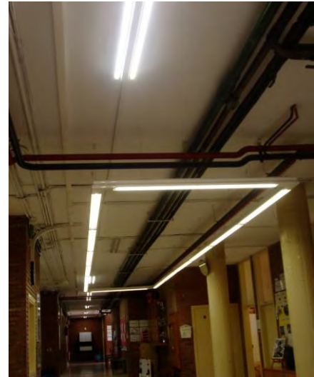
Figure 15- An illustration of how natural lighting should be complemented by artificial lighting with regulation of artificial lighting luminance (left); LED fixtures that look like fluorescent tubes reduce the electrical consumption and the heat load (right)
