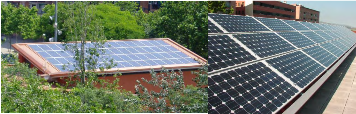
Figure 18- The photovoltaic modules installed on roofs have a high electricity production in Caribbean latitudes (versus PV on facades), besides, they reduce the thermal load from the ambient to the building if adequately ventilated
