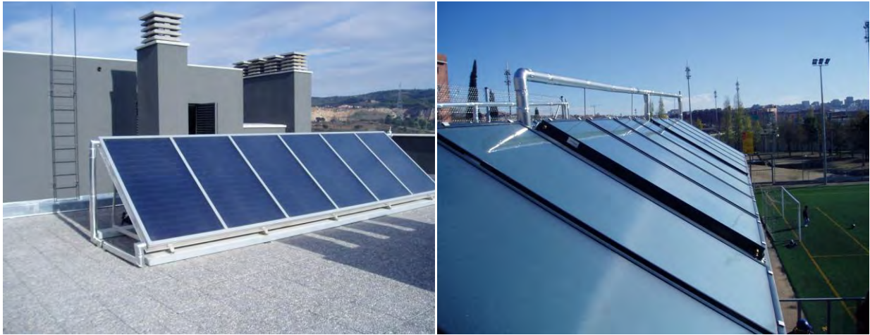
Figure 20- Service, commercial buildings (such as hotels, hospitals (right), sports centers (left) etc.) and residential buildings centralized solar thermal installations are the most effective solution to provide hot water all year round
