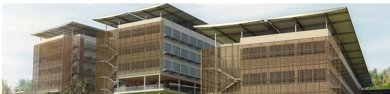
Figure 55- The EE Design incorporates a PV roof protected from extreme winds (top-left). In locations where extreme climatic events are weaker or non-existing, the PV itself can be a solar protection for the façade (top-right, bottom)
