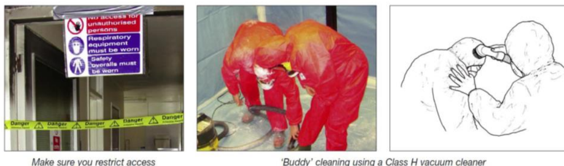
Figure 7.12.7: Asbestos Decontamination Practices [Ref. 67 ]
